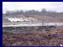
Picket dam, solids in front, lagoon in back
