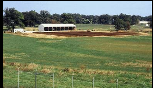
Compost Research Facility at Beltsville Agricultural Research Center
