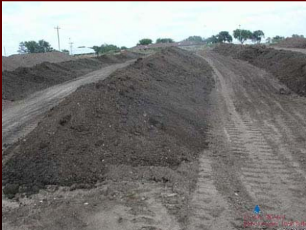
Dairy Manure Composting Facility in Erath County, Texas
